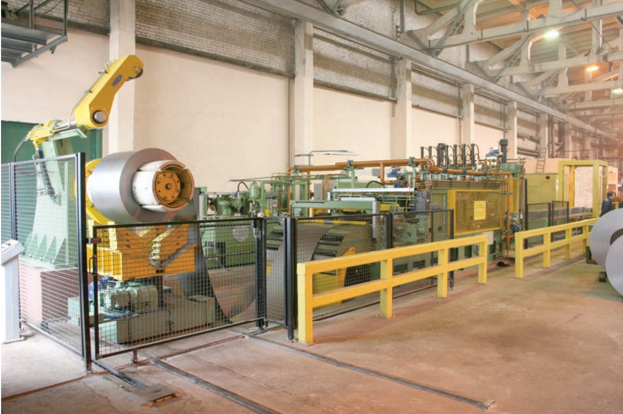
LINE FOR CORRUGATED WALLS OF THE TRANSFORMER TANKS (BY GEORG COMPANY)
